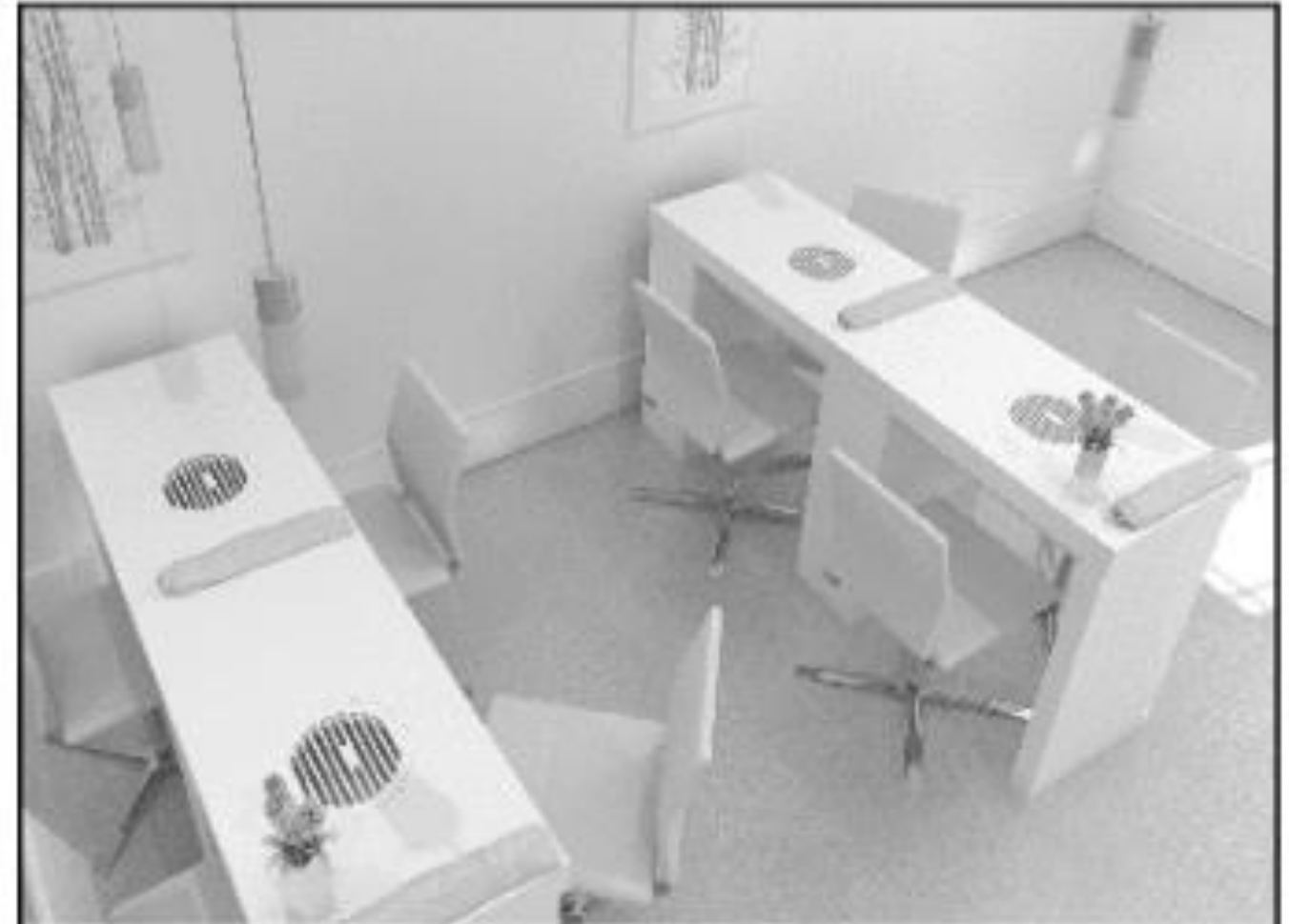
Commentary Figure 502.20.1(1) MANICURE AND PEDICURE STATION EXHAUST SYSTEM (Photo courtesy SalonSafe LLC)
