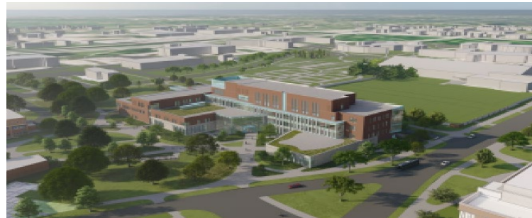
Engineering Design and Innovation Center
