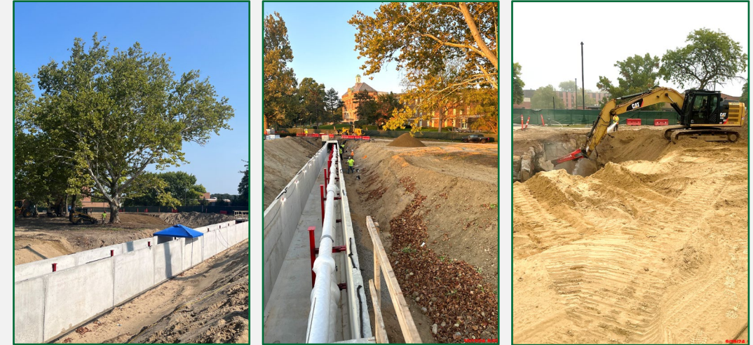
Jones Goddard Demolition Activities
