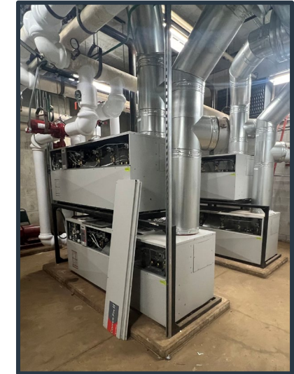
Boiler Replacement Project
