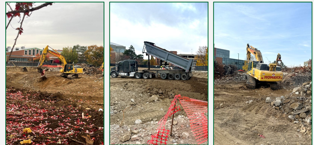
Brown Munson Demolition Activities
