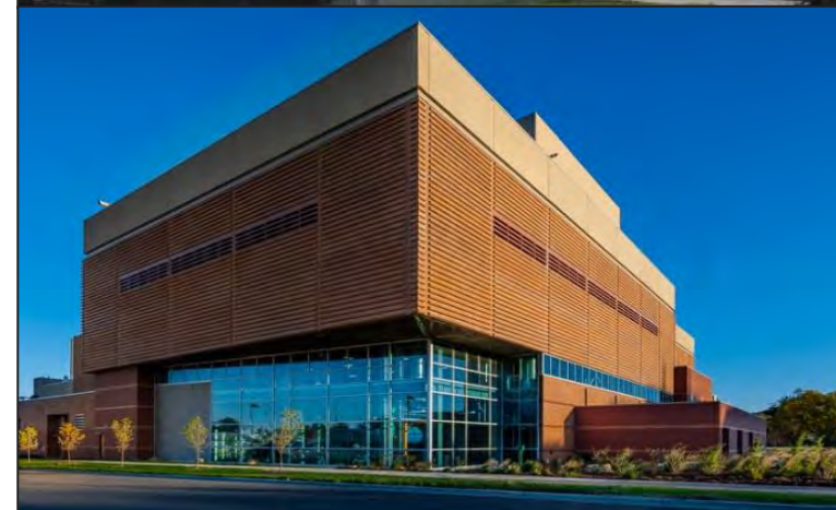
West Campus Cogeneration Facility
