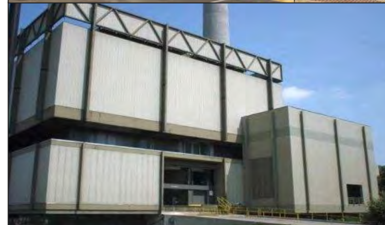
Walnut St H&C Plant
